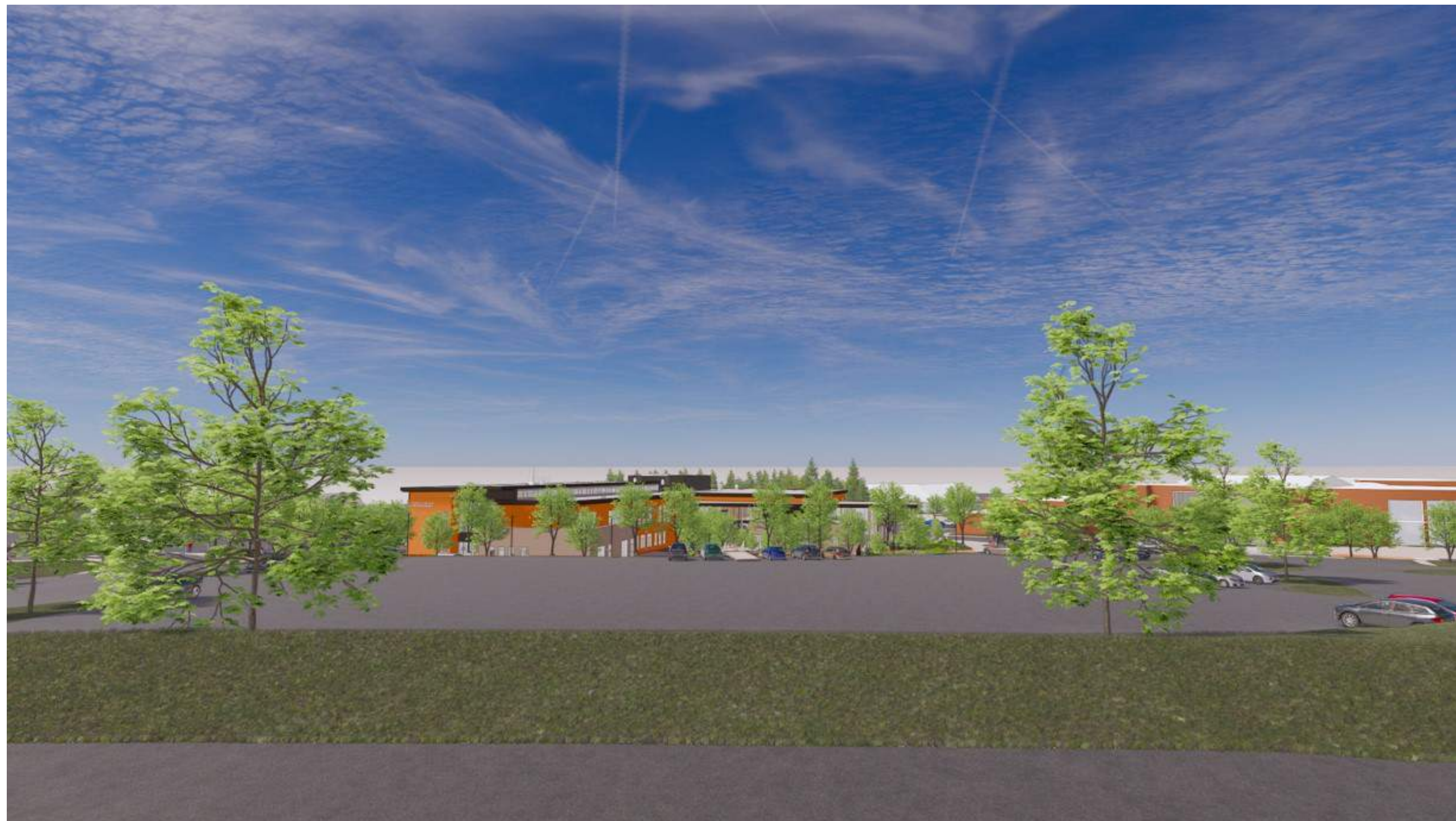
VIEW - FROM HYDRAULIC ROAD TOWARDS HIGH SCHOOL CENTER II MAIN ENTRY
